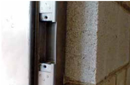
2. HES electric strike uses standard cutout
