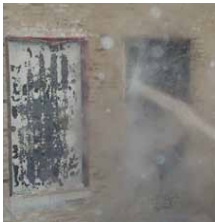
11. Applying water pressure
